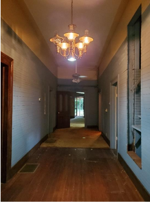
Figure 12 Overview of interior from corridor. Attic stair to right of photo.
