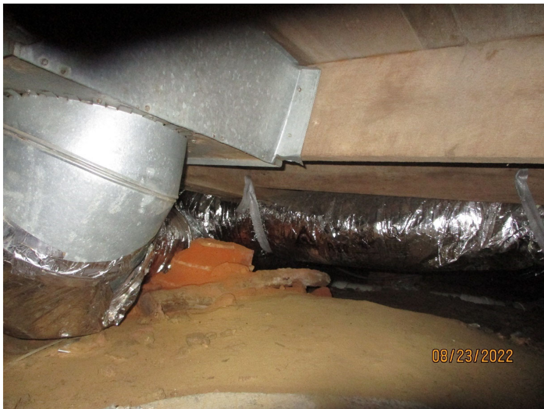
Collapsed foundation(6) below hallway wall
