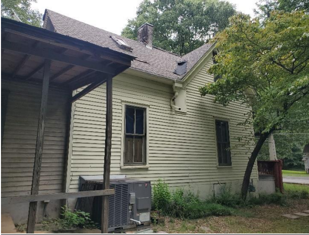
Figure 2 South side of house showing additions
