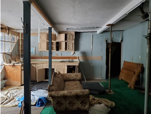
Figure 24 attic living room/kitchen showing temporary metal roof supports
