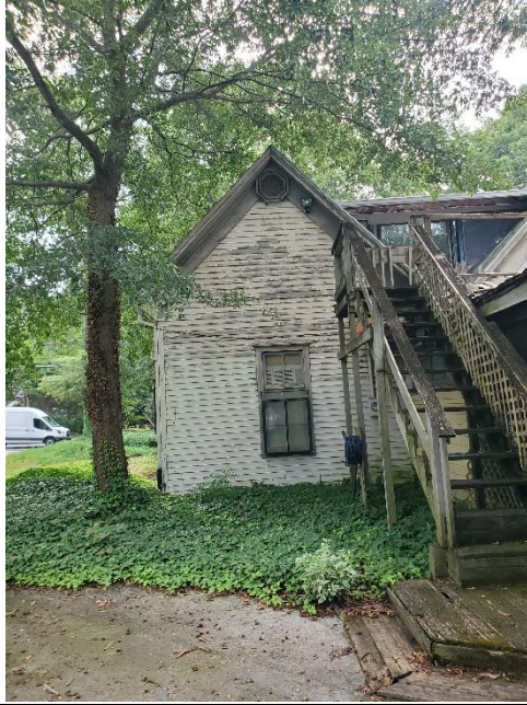
Figure 4 Rear of house showing deck stair and dormer installation
