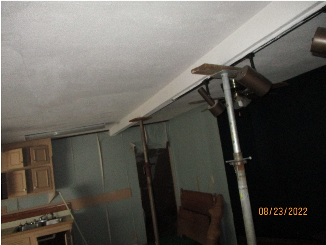
Roof support at upper room addition
