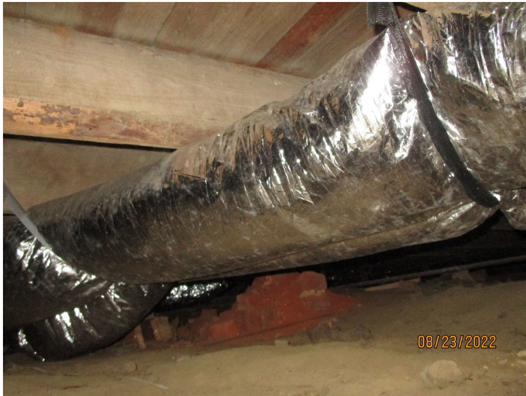
Collapsed foundation(5) below hallway wall
