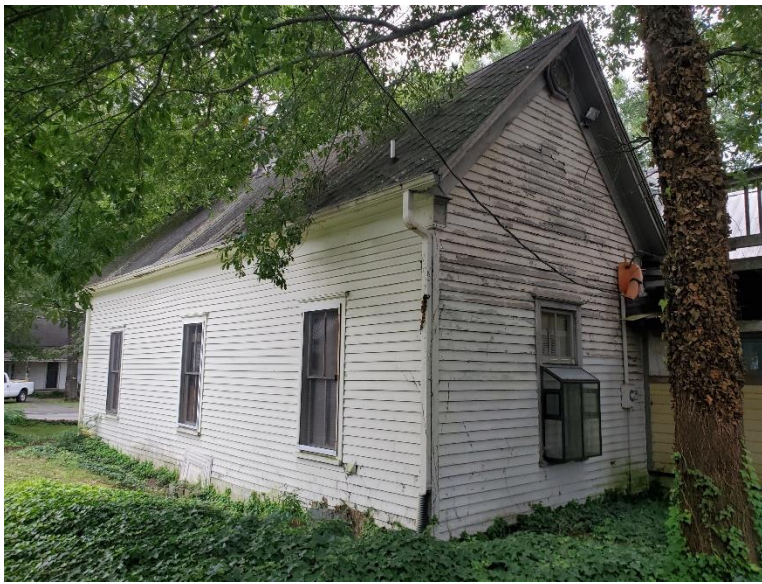
Figure 5 Side of house
