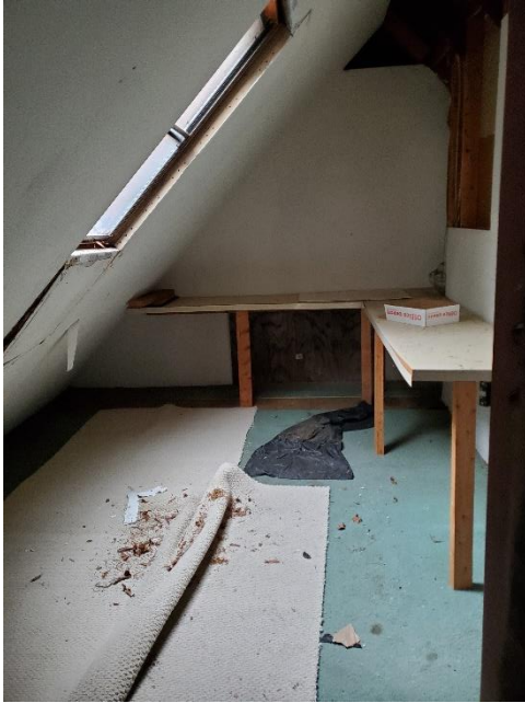
Figure 26 attic room showing skylight
