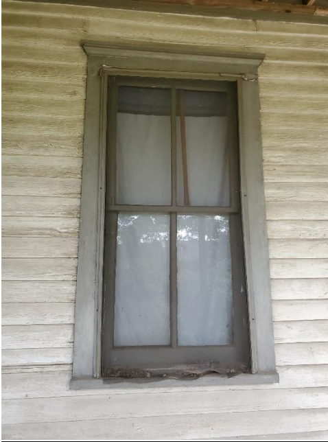
Figure 10 Original windows and trim
