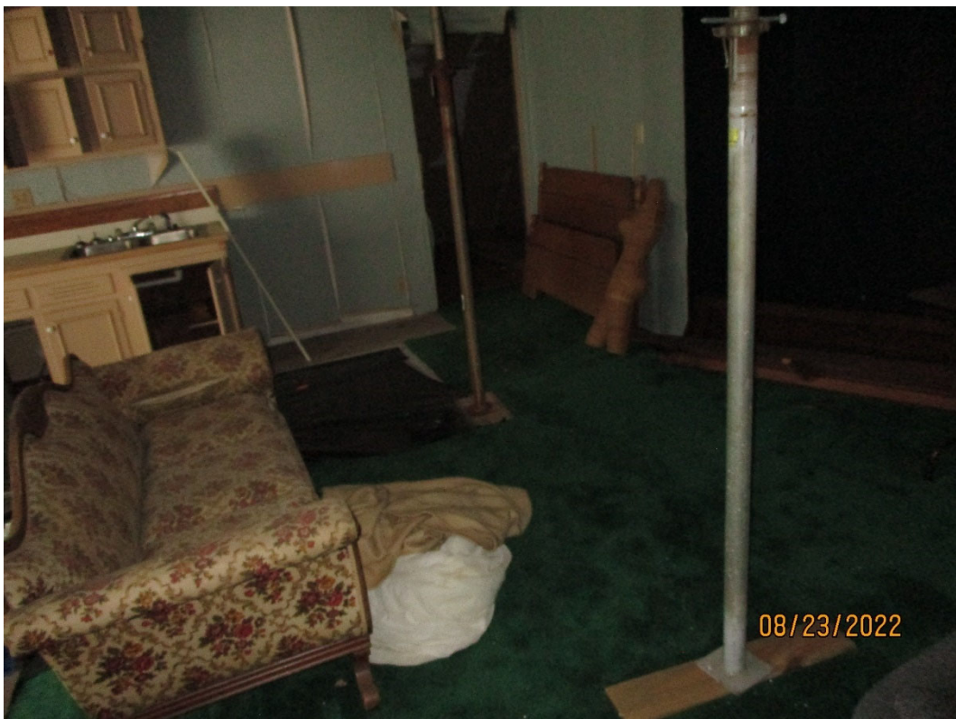
Base of post support for upper room roof
