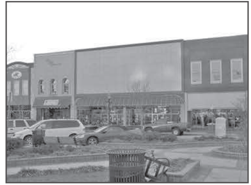
This storefront and upper floor in Gainesville, Georgia, has been inappropriately remodeled so that the original entrances have been lost and the upper floor windows have been obscured.
