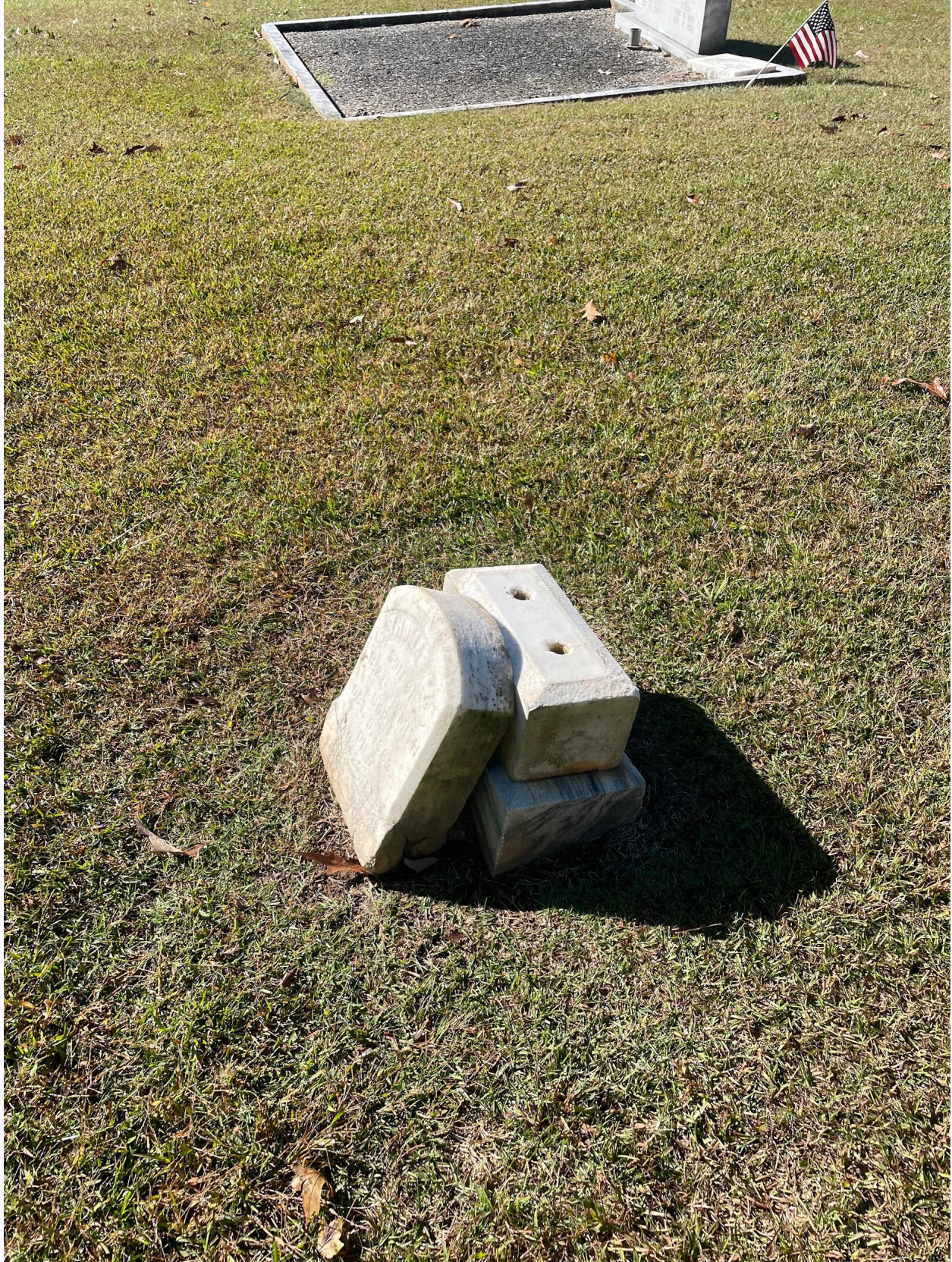
6. Infant reset + replace pins + point both levels w/ lime mortar - $125
