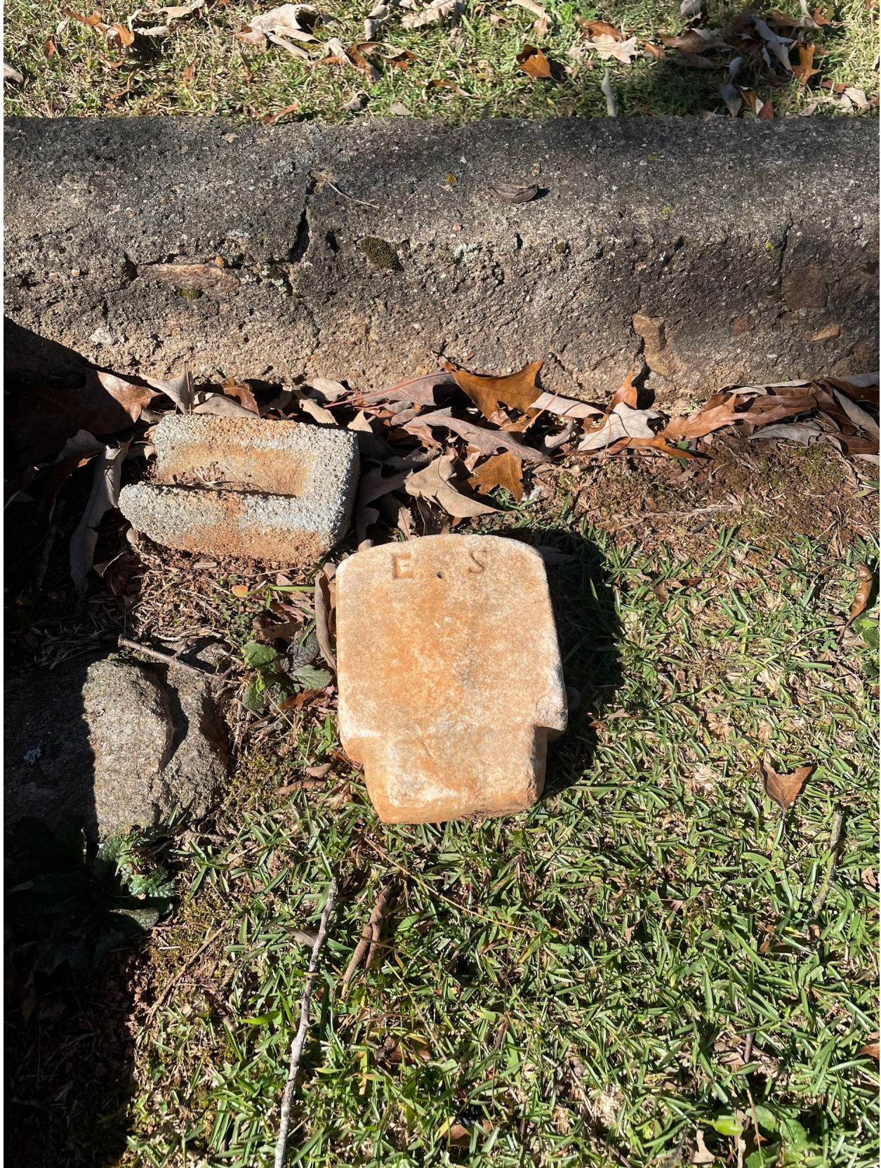
7. Make concrete socket + reset w/ lime mortar - $125
