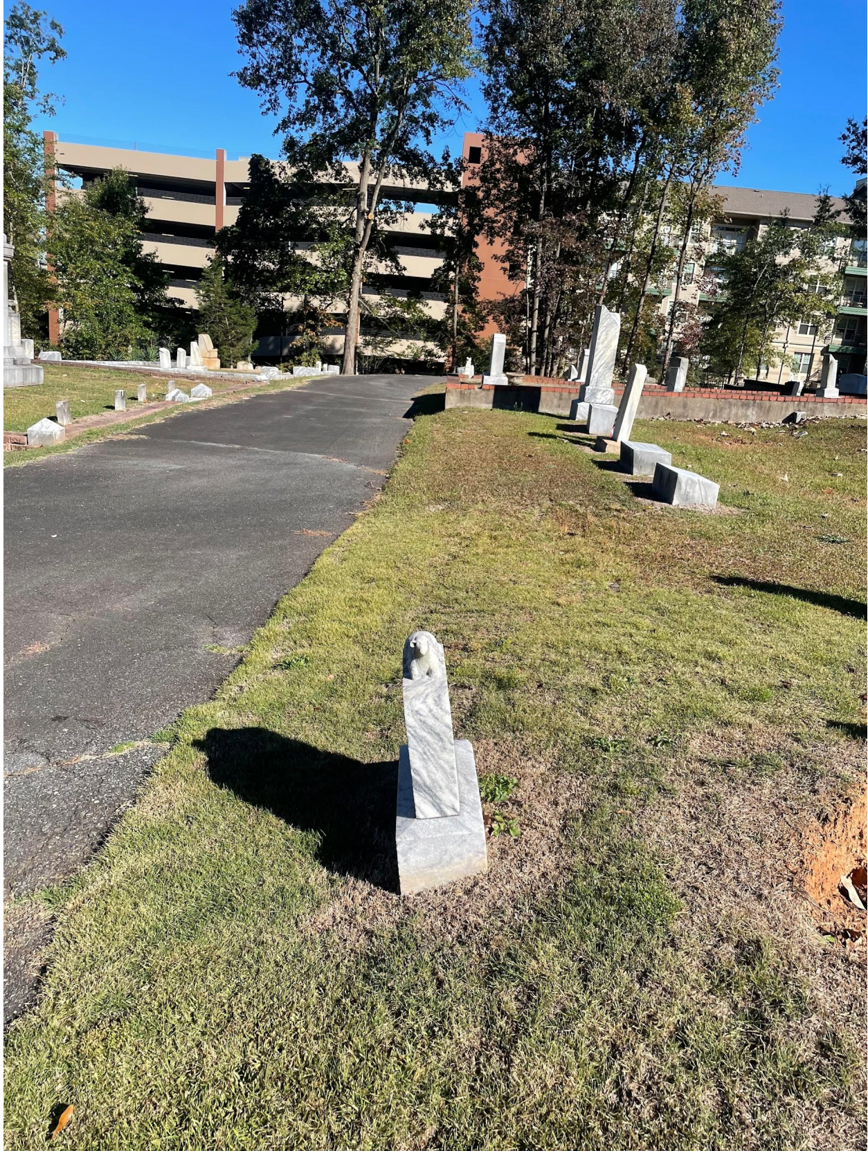
4. Concrete foundation + reset w/ lime mortar - $225
