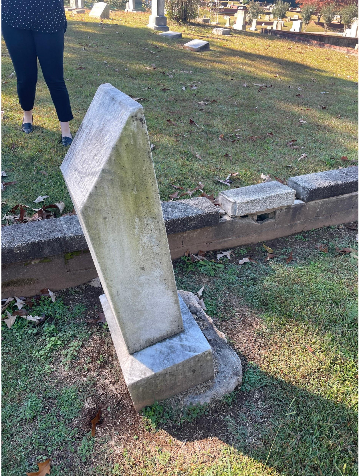
9. Priority* Remove old base, reset w/ 89 stone + point w/ lime mortar - $150
