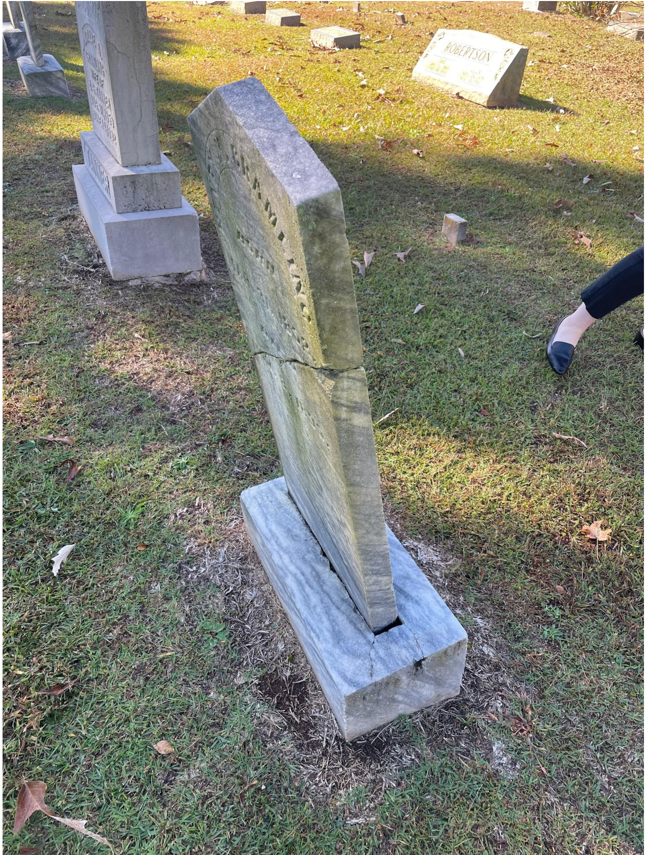
8. Priority* (large monument - helper needed) reset w/ lime mortar - $200
