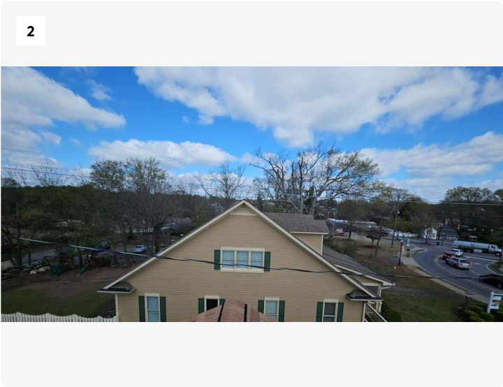
Left Elevation side of building showing the gable cornice returns on the End.
