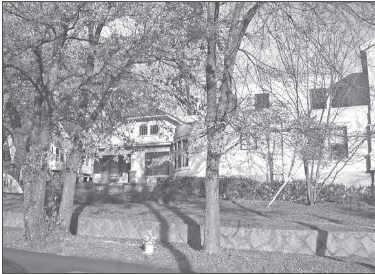
This clipped roof Bungalow in Stone Mountain, Georgia, was inappropriately rehabilitated for office use circa 2000. Inappropriate alterations include: 1) stucco was applied over the historic cladding of the original home; 2) the front porch was infilled; and 3) an addition double the size of the original house was added to the side and stepped forward in front of the original front facade.
