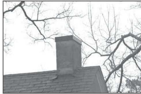
This interior chimney is covered in stucco. Stucco shall never be applied to a masonry chimney unless it was a historic feature of the building. If stucco was originally on a chimney it must be maintained.
