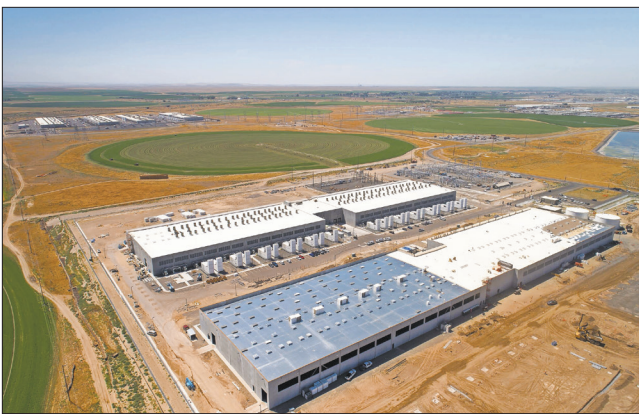
Dave Killen/oregonlive.com/TNS An aerial view of an Amazon data center near Boardman, Oregon.
