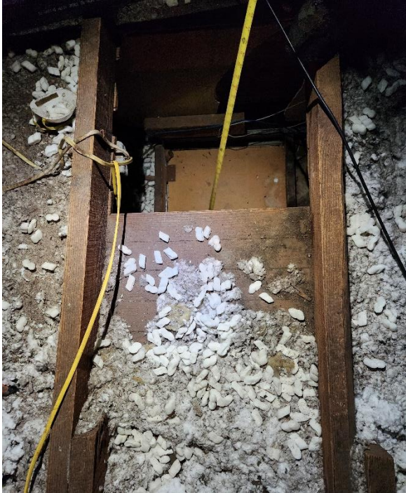
Figure 28 Attic framing showing minimal insulation, board ceiling, and lowered gypsum board ceiling below.
