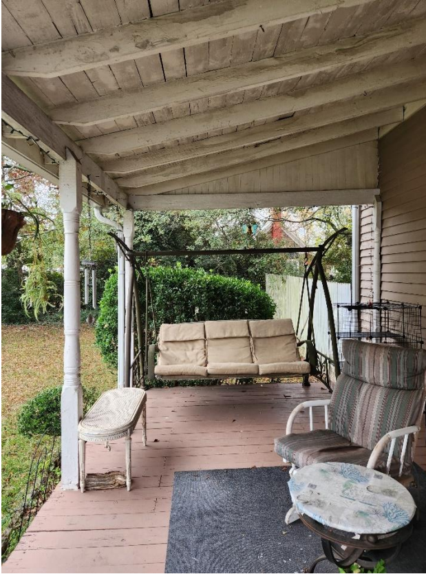
Figure 7 Front porch showing original turned columns, rafters and board ceiling and end boards. Decking is new.
