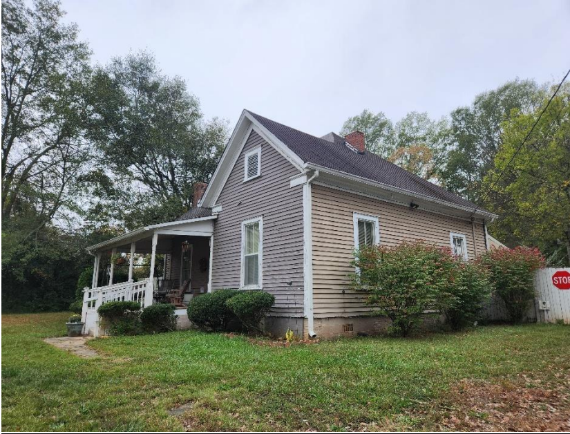
Figure 3 Side of house showing historic trim and chimney, siding, windows and porch
