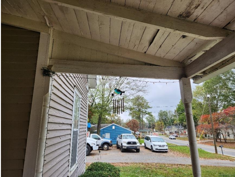
Figure 8 Original columns, ceiling, rafters, and bead board
