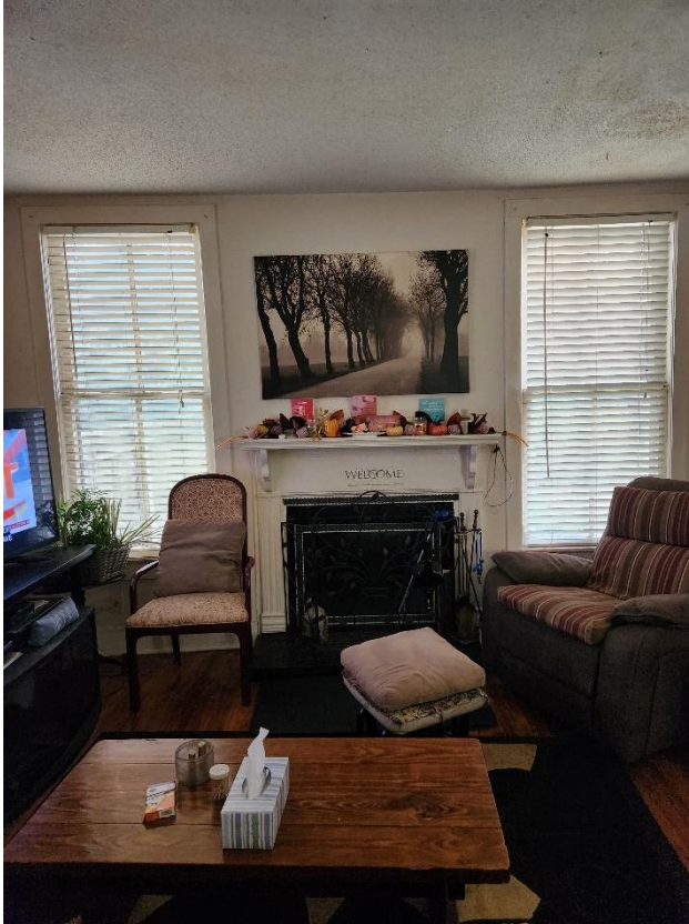
Figure 15 Living room showing original mantel and windows and dropped ceiling.
