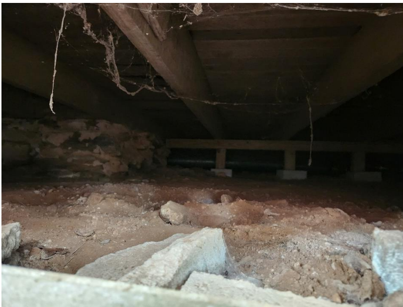
Figure 14 View of crawlspace showing original joists supplemented by an intermediate beam and posts
