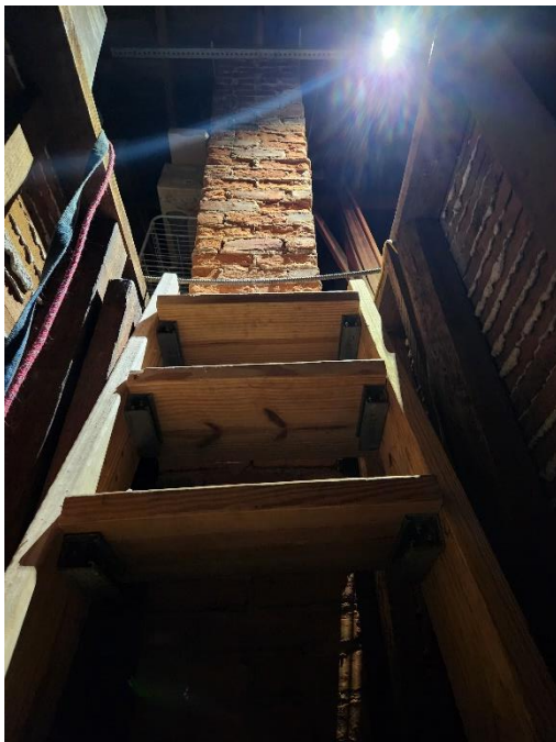
Figure 26 Attic access. Note plaster walls and spalling brick at chimney
