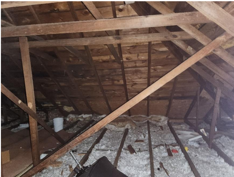
Figure 29 Attic framing showing cross-bracing and patch at corner.
