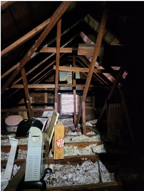
Figure 27 Attic framing at front gable
