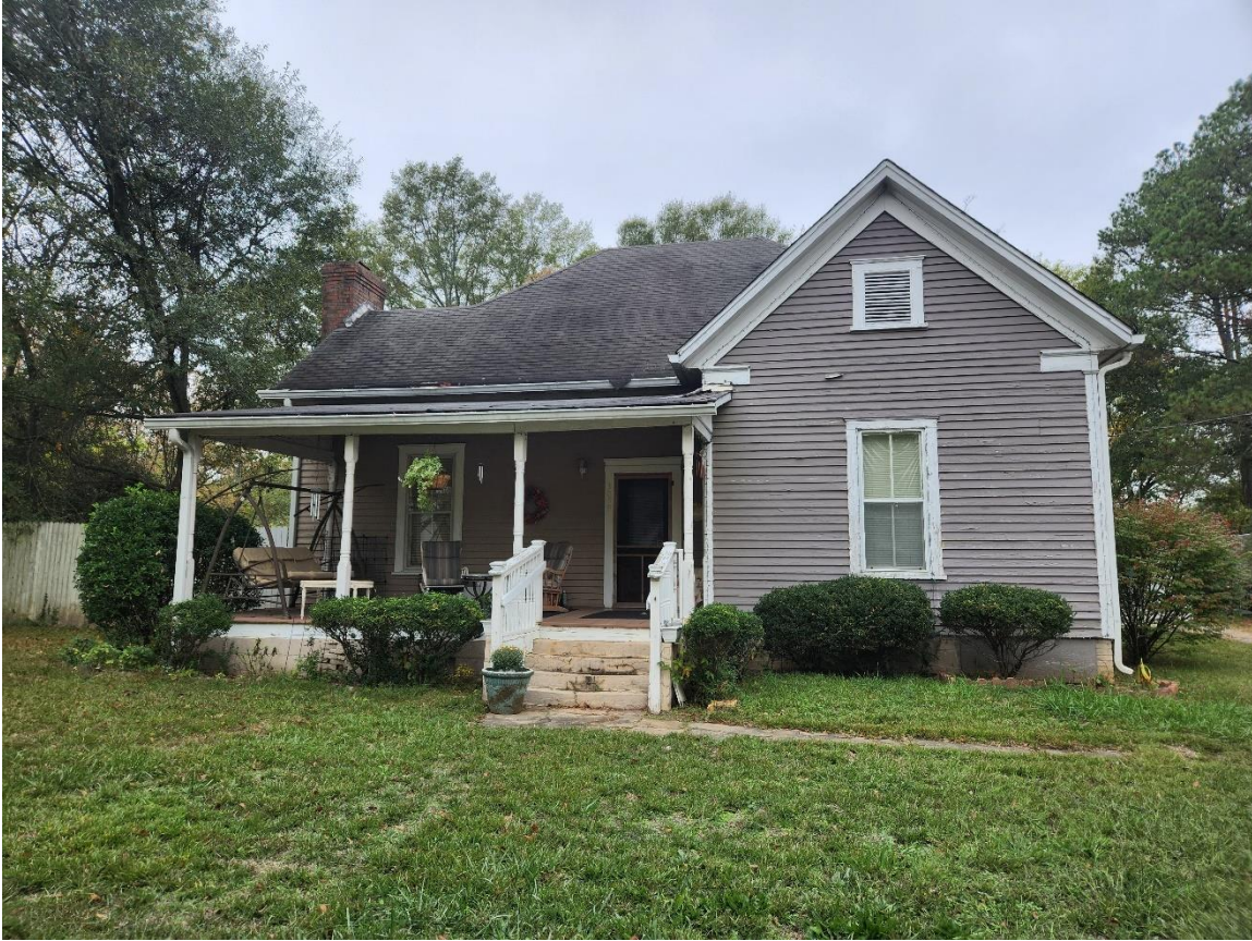
Figure 1 Overview of house from street
