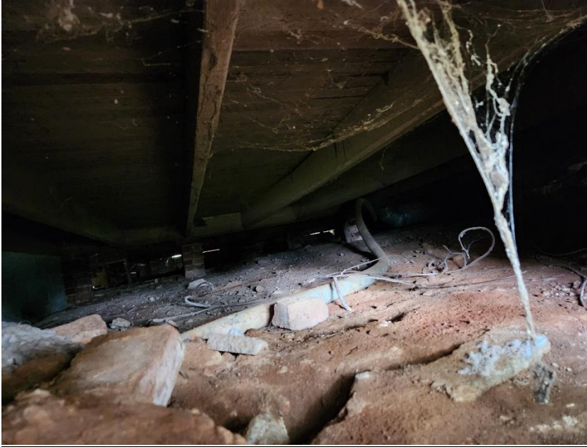
Figure 13 Foundation showing original joists. Very narrow crawlspace with limited visibility.
