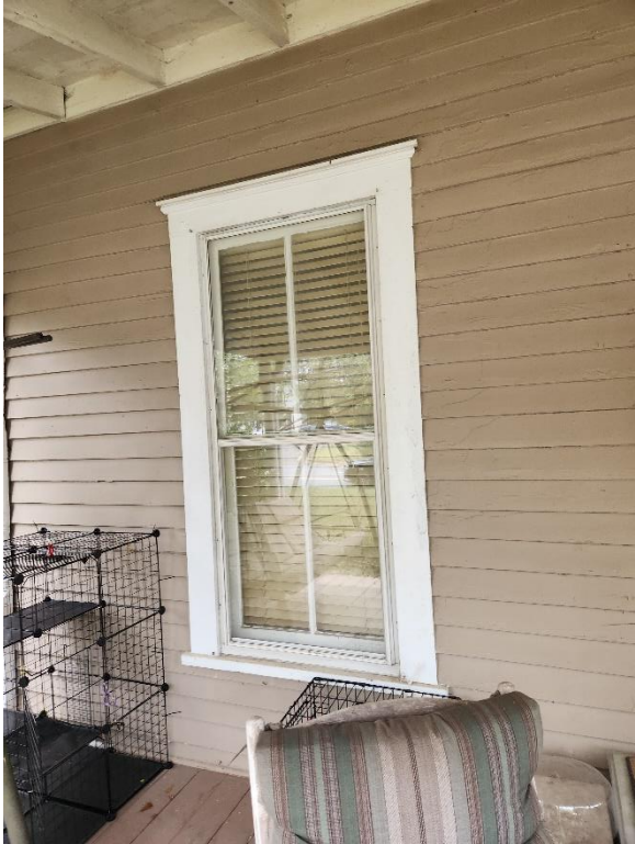
Figure 11 Original window and trim. Window covered by storm window.
