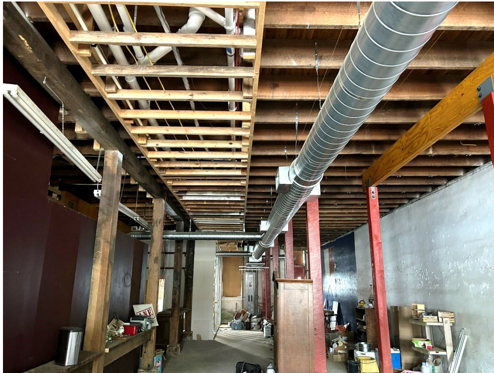
Ground floor interior
