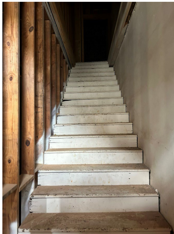
Ground floor rear stairwell
