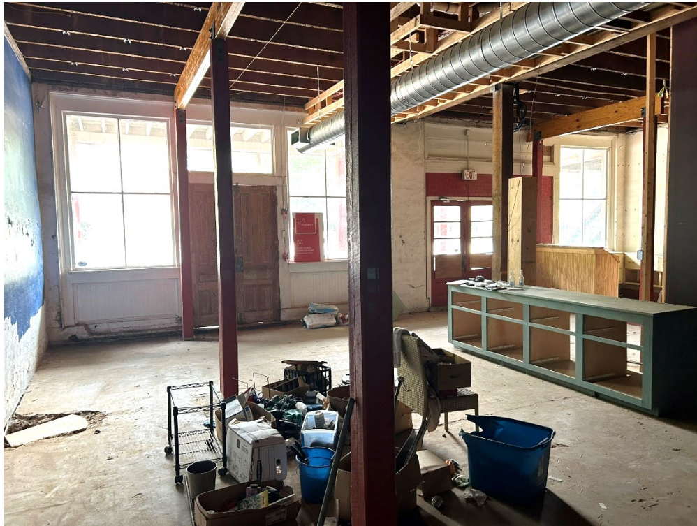
Ground floor interior
