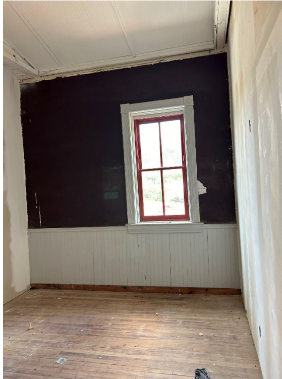
Third floor interior
