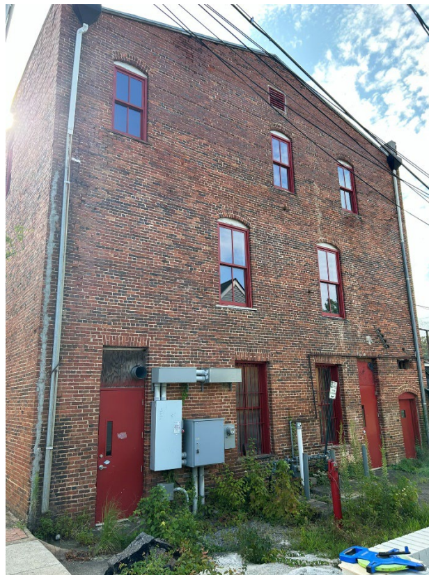
Rear view of Subject
