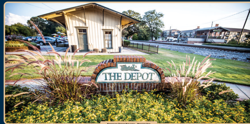
KENNESAW DEPOT BUILDING - PRESENT DAY
