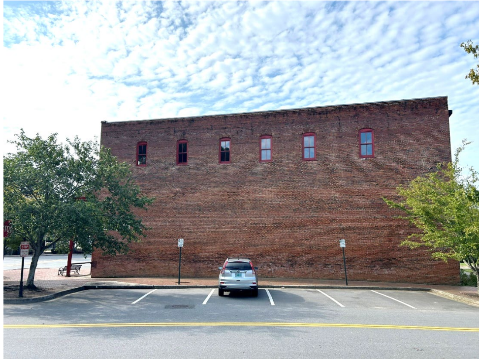
Subject's north wall along Lewis Street looking South
