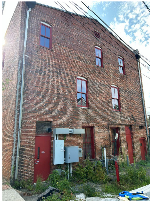
Rear view of Subject
