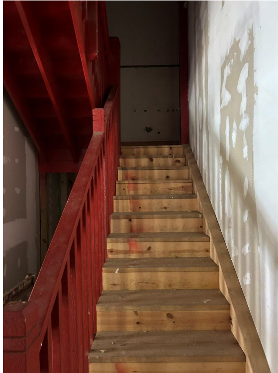
Ground floor front stairwell
