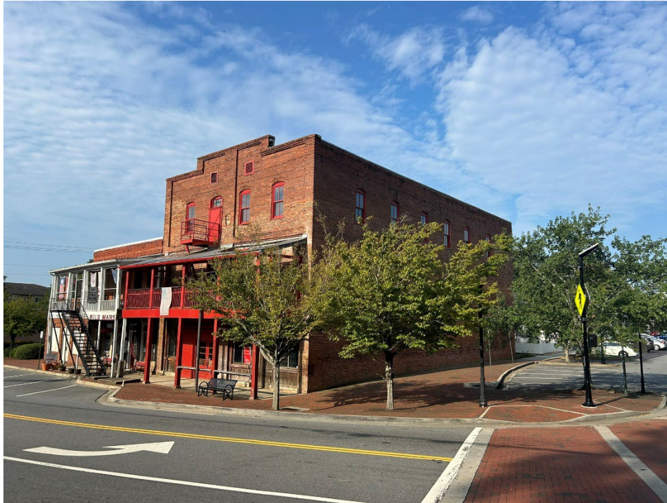
Subject frontage along North Main Street looking SW
